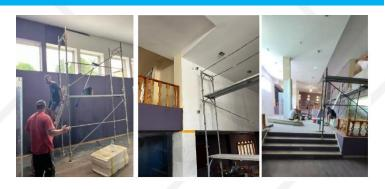
Damaged doors and windows were replaced to improve security and insulation, while the museum's cladding was updated with new boards for added protection and aesthetic appeal.
